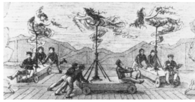
Fig. 4 The swimming machines (for Das Rheingold ) in action
